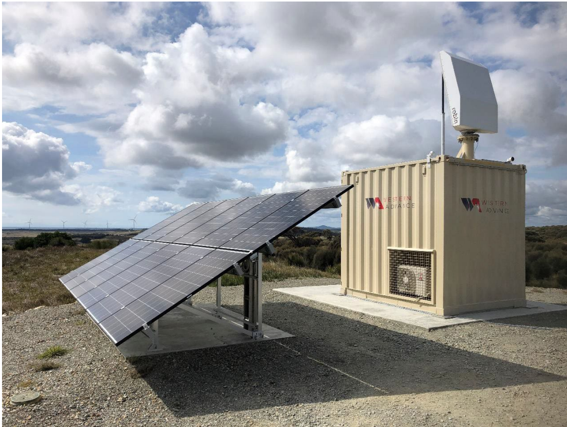
Figure 6. Installation and commissioning of the Robin Radar system was completed in October 2020. This included the back-up solar power supply and the lightning conductor mast in the background.
