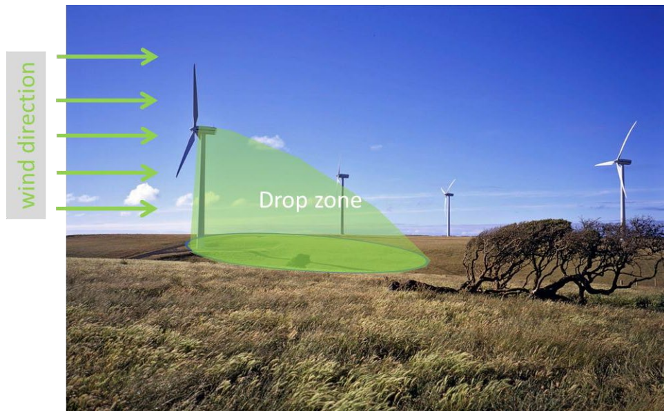
Figure 4. A further example of the extent of the drop zone under high wind conditions.
