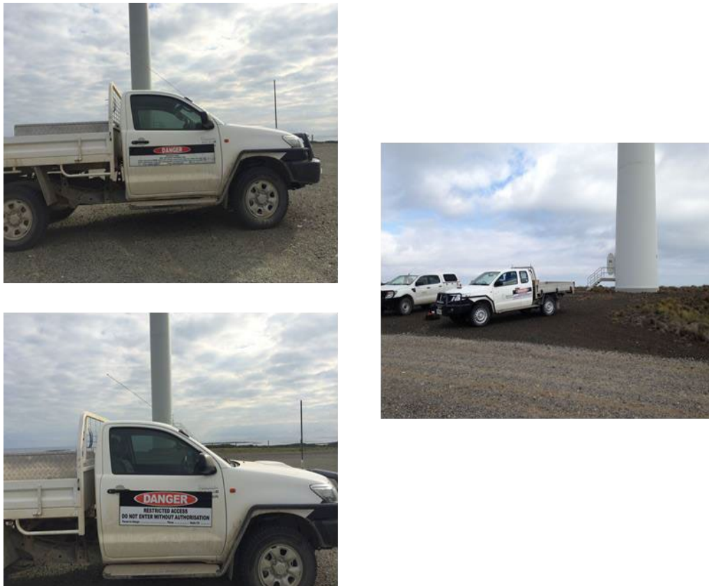
Figure 6. This sign, or similar, shall be placed in a suitable location to ensure the drop zone is identifiable.
