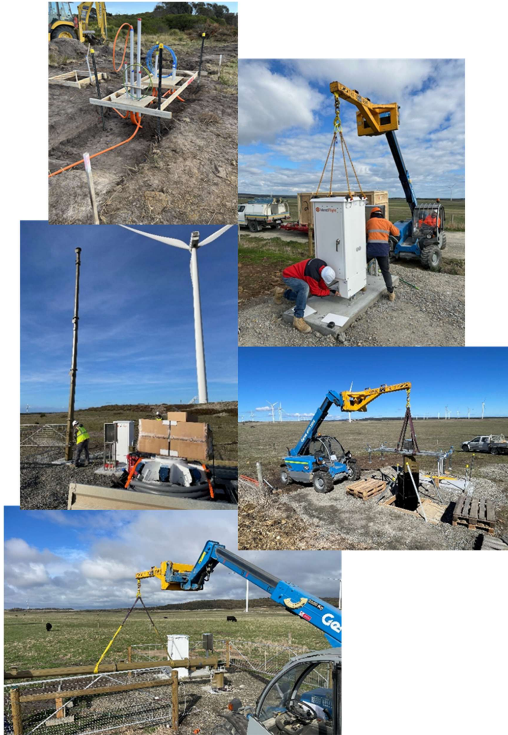
Figure 6. Photos from the construction and installation of the IdentiFlight system at MRWF. Clockwise from top shows the conduits positioned prior to the slab being poured for the control cabinet at each IdentiFlight tower, the installation of the control cabinet, a telehandler carefully lowering the embedded tower section prior to pouring the concrete footing, the tower being positioned ready for bolting to the embedded section, and final standing of the tower ready for the attachment of the imaging head by IdentiFlight technicians.
